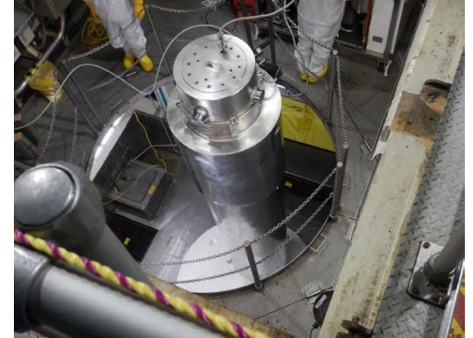
Above: Technicians at Dominion Virginia Power's North Anna nuclear plant prepare a shipping cask containing fuel rods from HBU assemblies for shipment to ORNL. http://eprijournal.com/spent-nuclear-fuel-storage-demo-heats-up/
